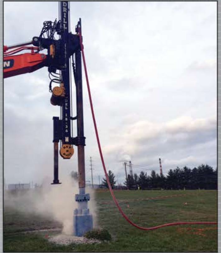
The LP drill on a small excavator mount.
